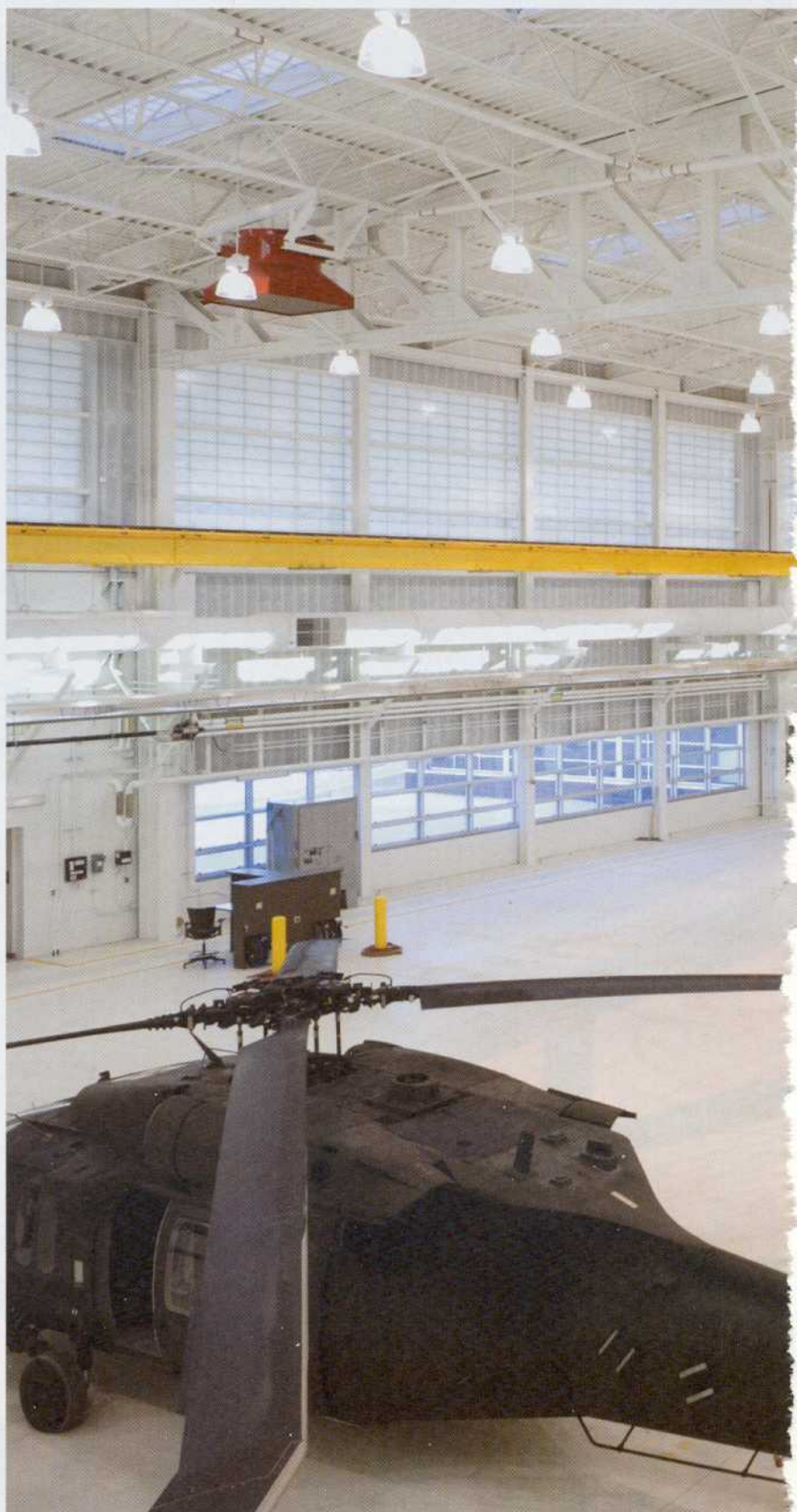
Above: Clerestory windows and skylights provide plenty of daylighting inside the hangar. Left top: An exterior rendering shows the landscape plan that includes native plantings. Left above: The building's graceful form is brought into focus after a snowstorm.
